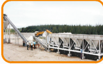
Wet Mix Plant
